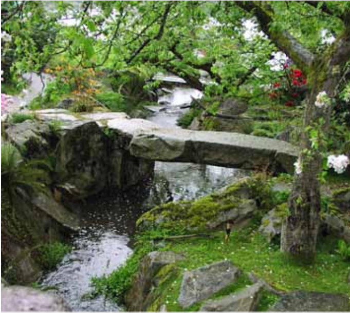
Griffith Slab Bridge: Transformation of a gully into a naturalized rock-lined creek that provides ideal salmon spawning habitat – Mercer Island, Washington.
