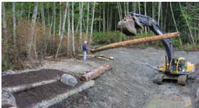
Lake & Wetlands Completion: Thriving wetlands habitat, well established and performing as nature herself created it, in just 8 months.
